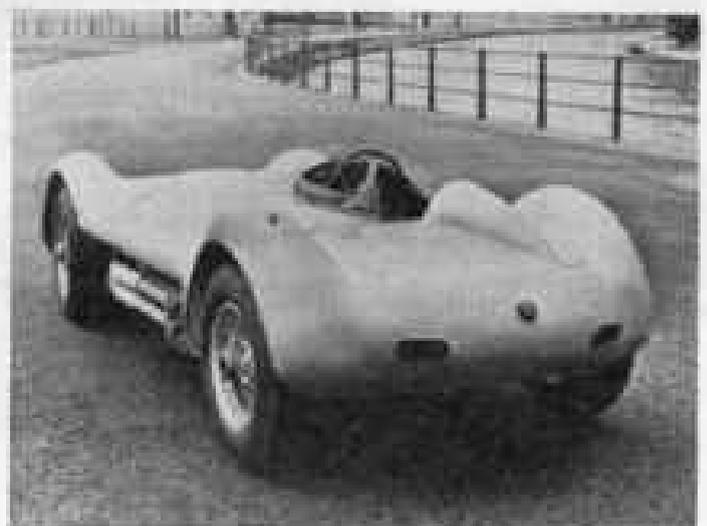
*Rear view shows hot air outlets for inboard disc-brakes and differential unit. There is room for driver's head under passenger seat panel in the event of turning over.*
